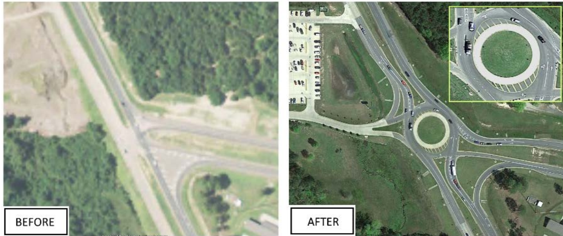
FIGURE 10 Before-and-after images of LA 8/28 at US 171 intersection.
