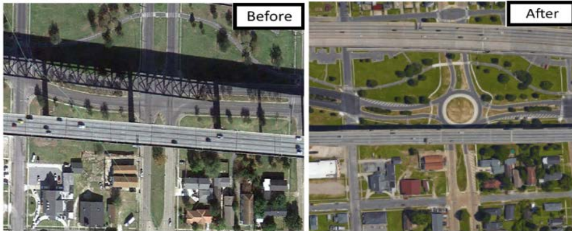
FIGURE 13 Before-and-after images of LA 428 at Mardi Gras Blvd. roundabout.
